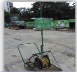
Reuse of waste metal as dust suppression facilities
